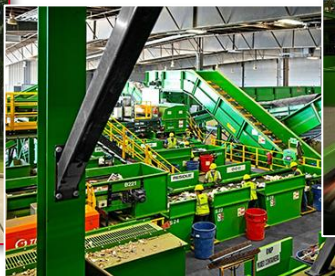
WM Waste processing in Orange County
